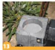
13 Thermoweld system is ready for fire.
