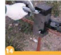
14 Fire the thermoweld igniter by the igniter gun.
