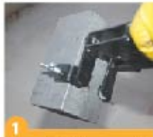
1 Connect the thermoweld mould with thermowelding plier
