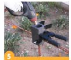
5 To prepare for heating inside of the mould
