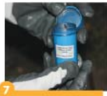
7 Open the lid of the thermowelding box
