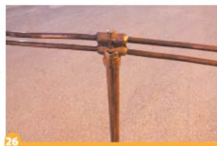
Welded earthing conductors and earthing electrode.
