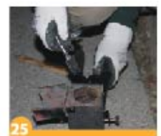
25 Clean the mould for new application
