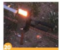
20 Thermowelding has finished
