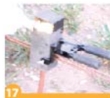
17 Thermoweld powder fired.
